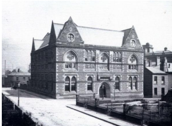
Figure Three – Historical image of the site (c 1880)
